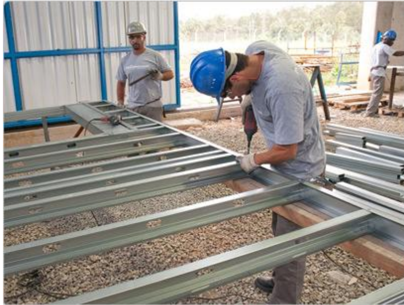
Figura 12: Painéis Steel frame
