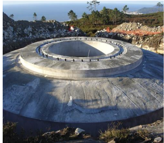
Figura 19.3 – base concretada
