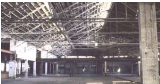
Interior of Market Hall Prior to Restoration
