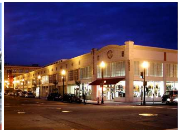
Original 10th Street Facade
