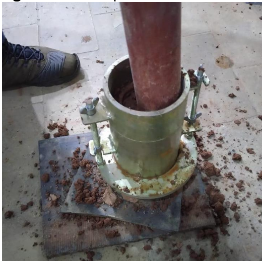
Figura 21: Compactando as camadas
