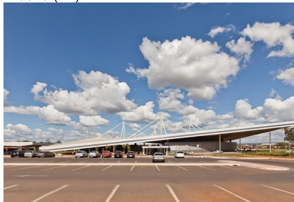
Figura 43 – Vista lateral/ Terminal Rod. de Brasília (DF).
