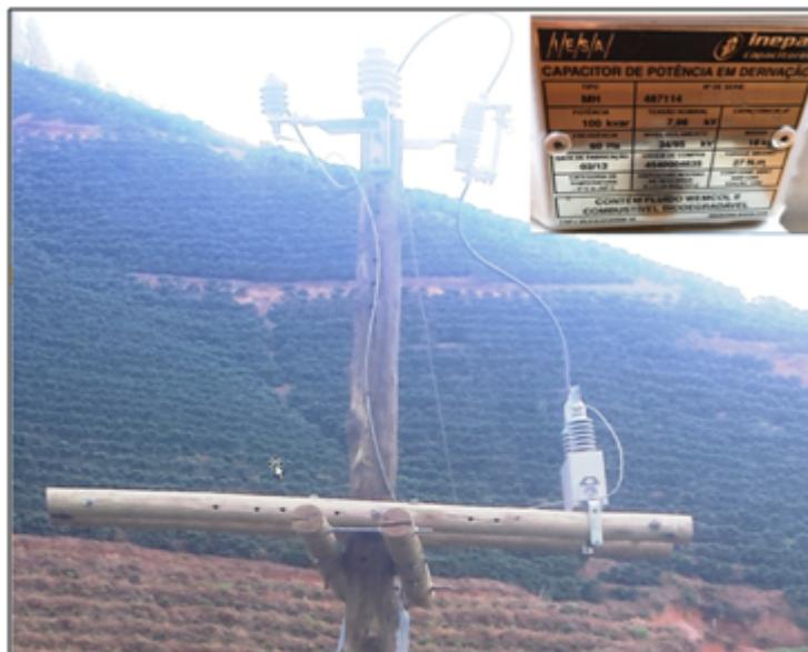
**Figura 16:** Capacitor instalado
